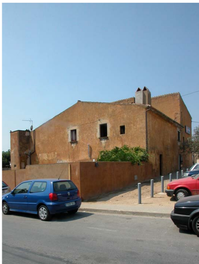
CARRER FITOR Nos 1-3
